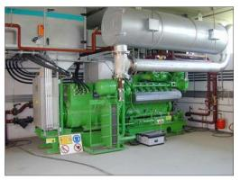
The Landfill Gas to Energy Facility began operation in 2012 and consists of 4 GE Jenbacher Engines which produce 4.2 MW of electricity, powering approximately 4,000 homes.
