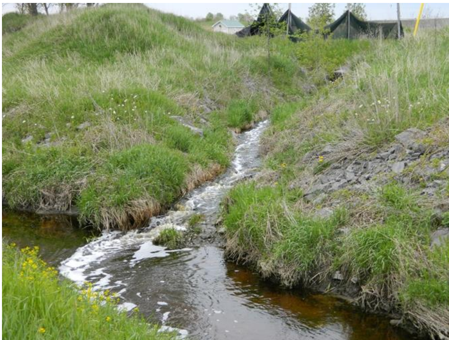
Photograph 4 View of Treated Effluent Discharge Stream entering Fraser Drain (2019-05-23)
