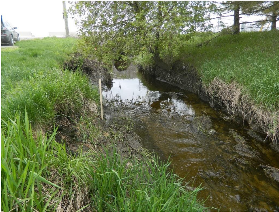
Photograph 3 Looking upstream at SWFD3 toward Laflèche Road culvert (2019-05-23)
