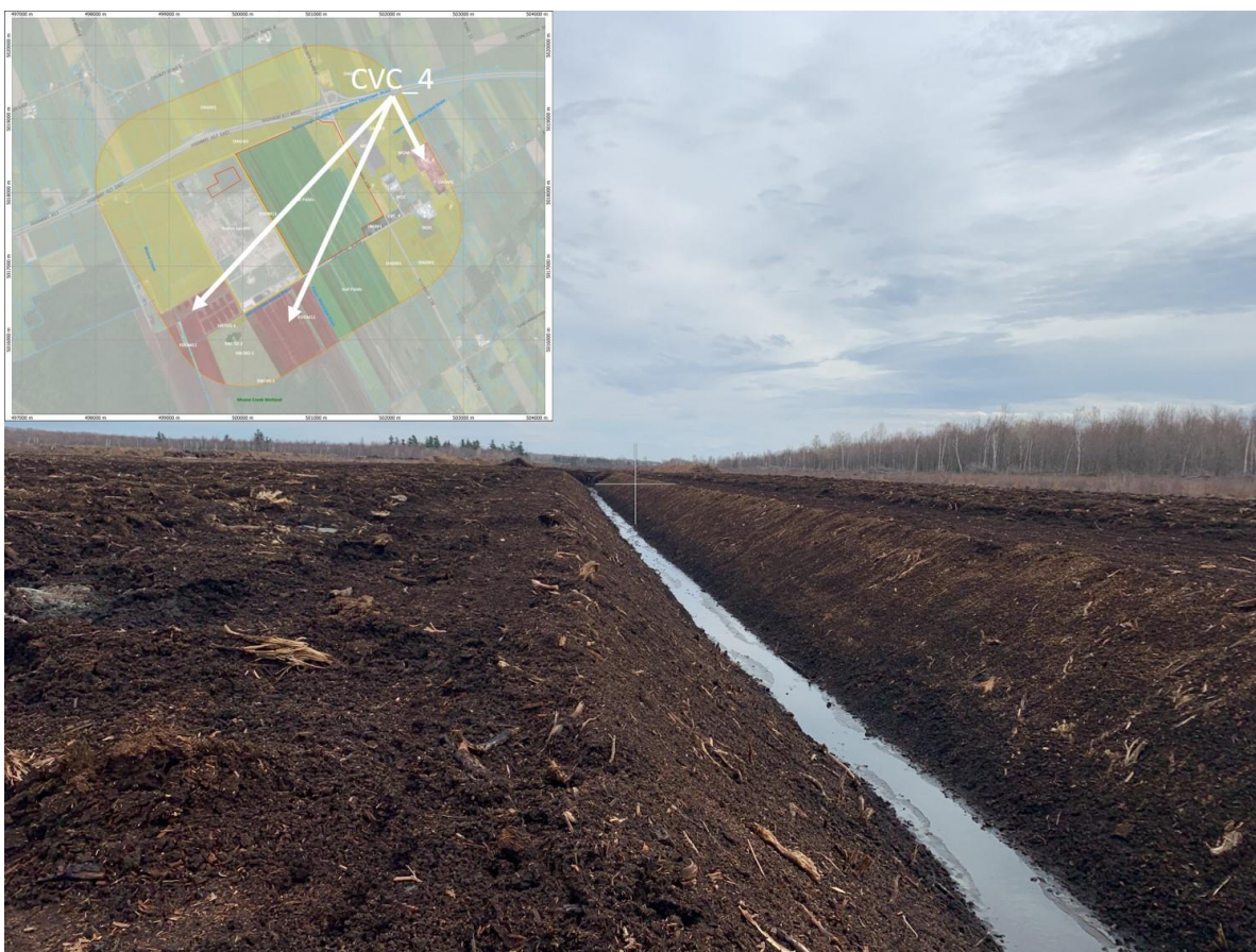
Figure 13 Photo showing peat excavation operations (CVC_4) off-Site taken April 23, 2019
