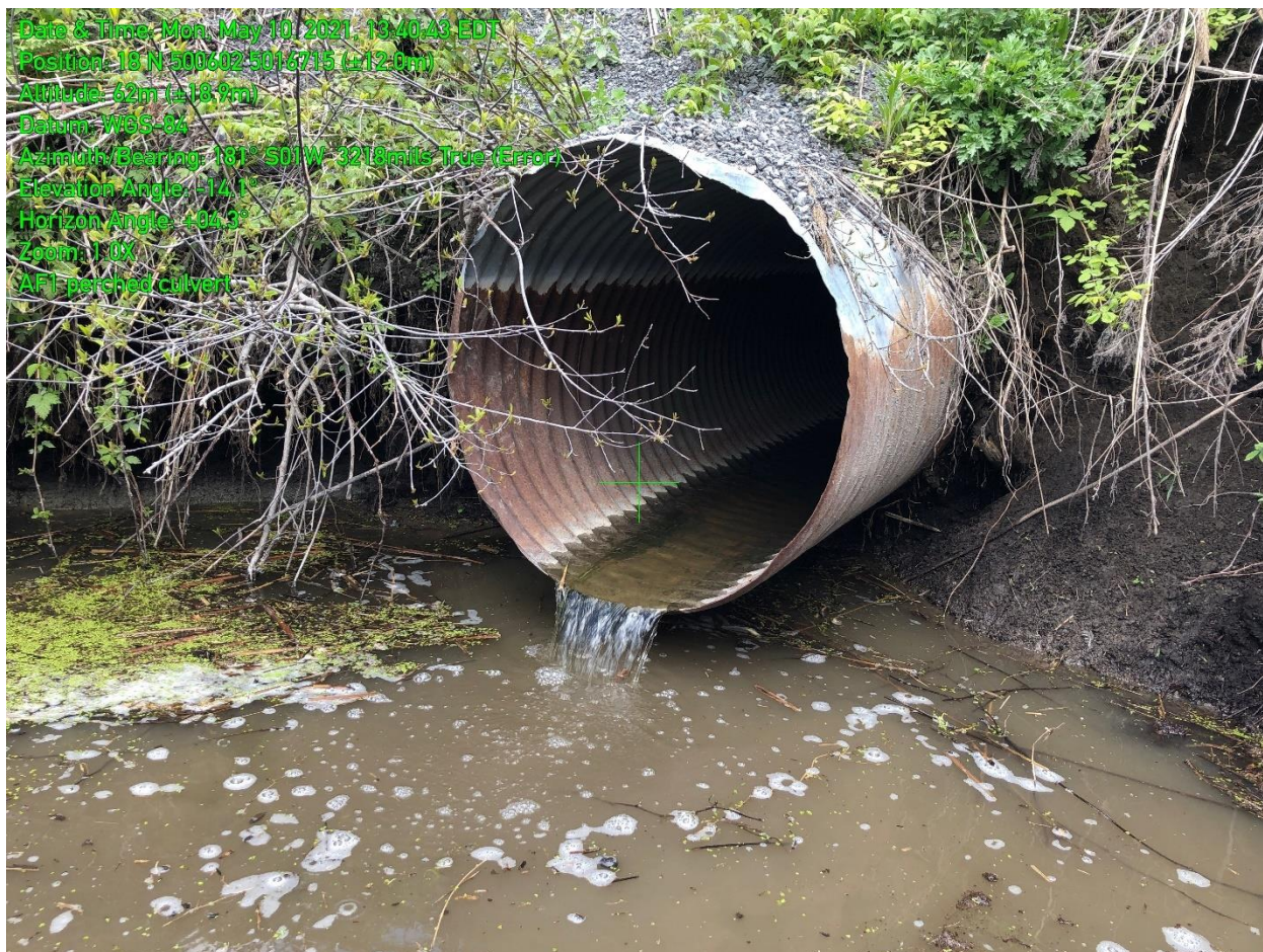
Figure 19 Photo showing the perched culvert near the upstream end of the Albert Fahey Award Drain at electrofishing station AF1 taken on May 10, 2021
