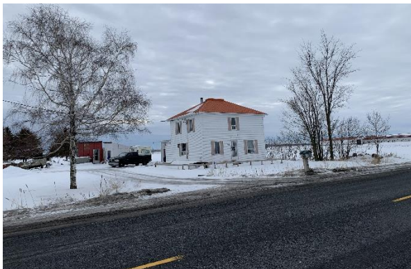
Looking southeast towards the residence at 1790 County Road 8 (ASI 2019).
