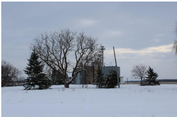
Looking southeast towards industrial farm structures across agricultural fields towards the farmstead (ASI 2020).
