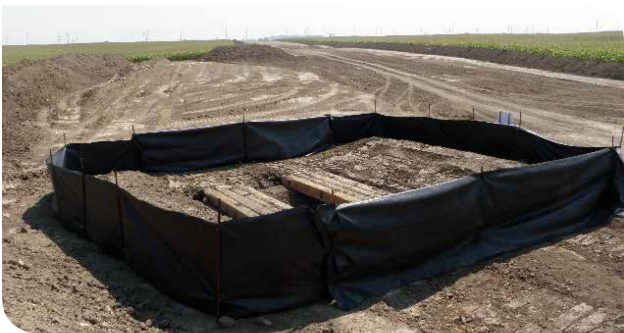
Cleaning station at construction site.
