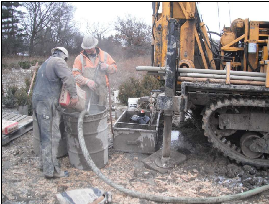
Photograph 2.2-6 Mixing bentonite grout prior to pumping it into piezometer annulus
