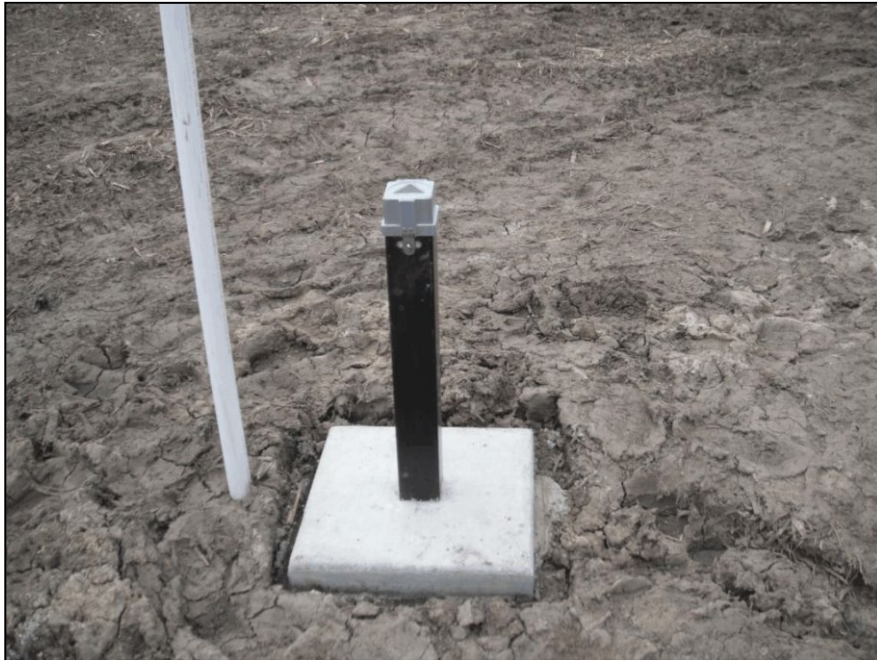
Photograph 2.8-1 Typical Monitoring Well
