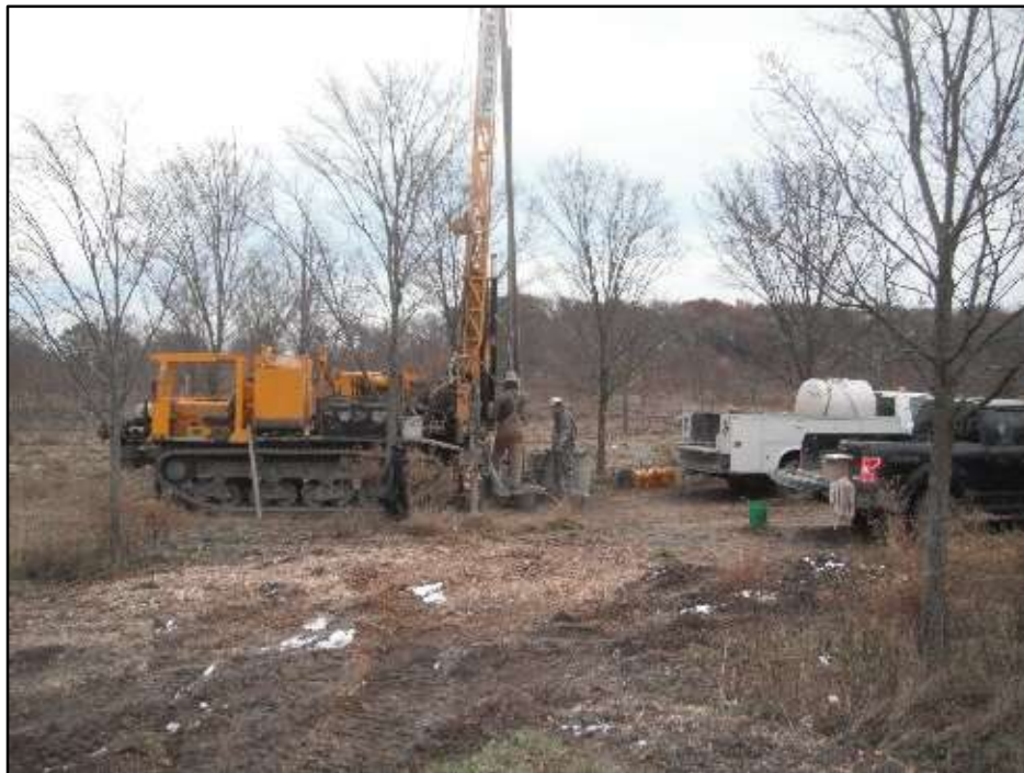
Photograph 2.2-1 All-Terrain Drill Rig
