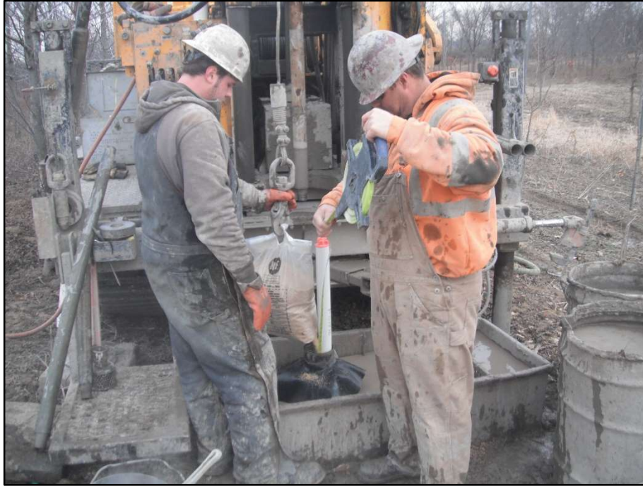
Photograph 2.2-4 Installation of sand filter pack
