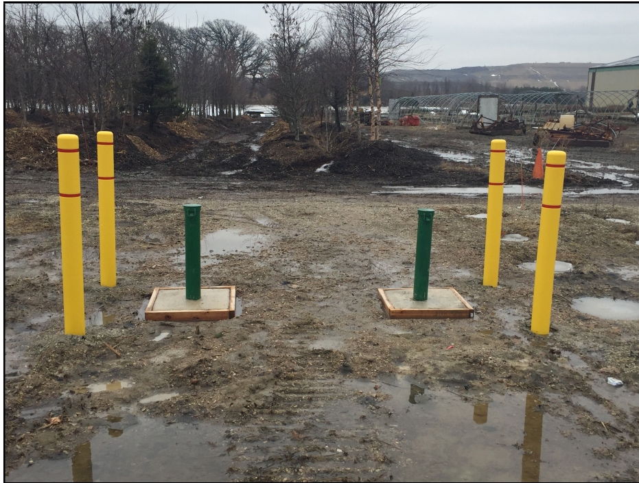
Photograph 2.2-7 Finished piezometer cluster at boring location B-14-18
