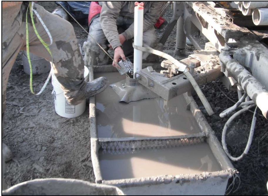
Photograph 2.2-5 Installation of bentonite pellet seal
