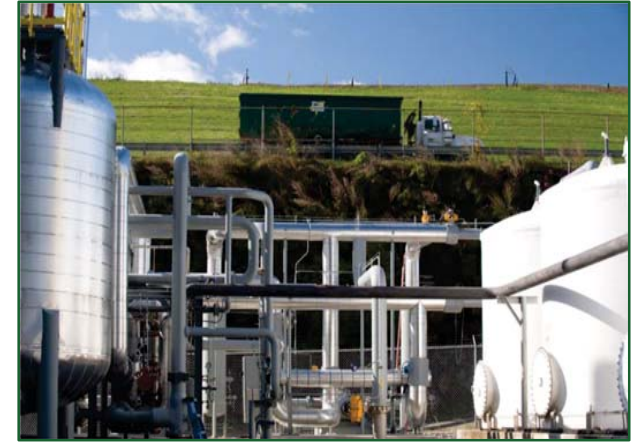
High-Btu Pipeline Project Rochester, NH
