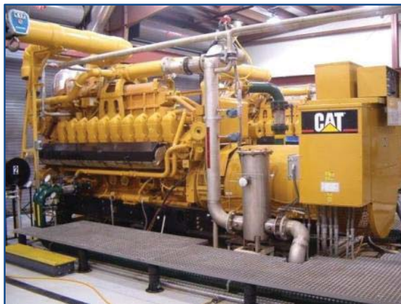
Internal Combustion Engine (range from 100 kW to 3 MW)
