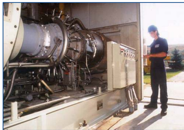
Gas Turbine (range from 800 kW to 10.5 MW)
